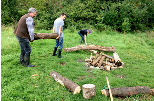
Hard at work replacing the fire pit seating
